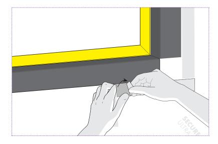
Once the previous step is complete, peel off the release liner from the Cortex® Double-Sided Tape. Some may prefer to remove the release liner as they adhere the membrane.
