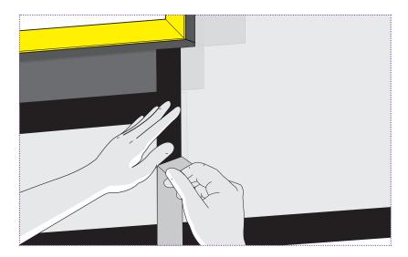
Finally, use the Cortex® UV Facade Tape to seal off all the edges.
